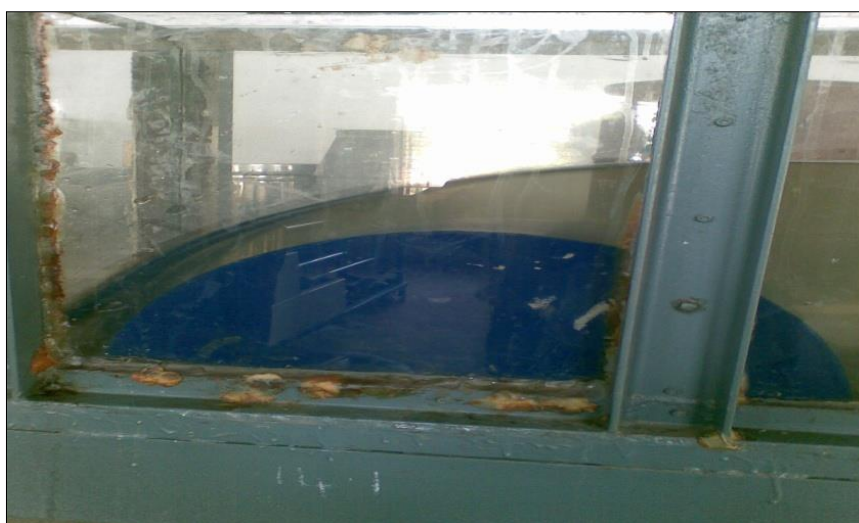
Fig 1: Installation of Circular Crested Weir
