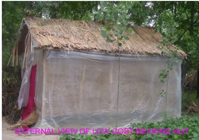
External view of Low Cost Rearing Hut
